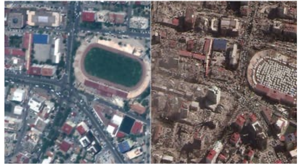
Turkey Earthquake 2023 Destruction [im1]
